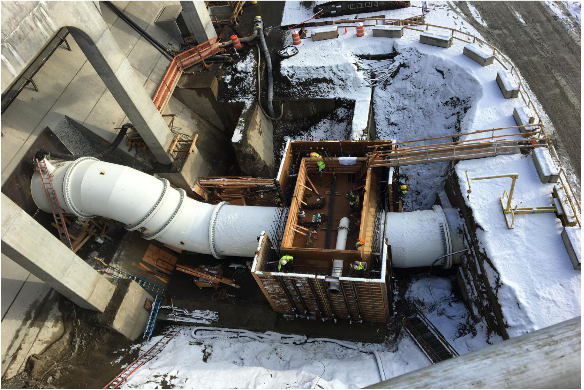
Construction of AWS 10' valve room.
